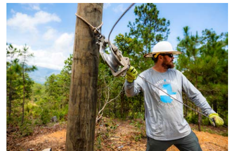
GVP lineman Zeb Birch is hard at work bringing first-time light to rural Guatemalan village La Montanita de la Virgen.
