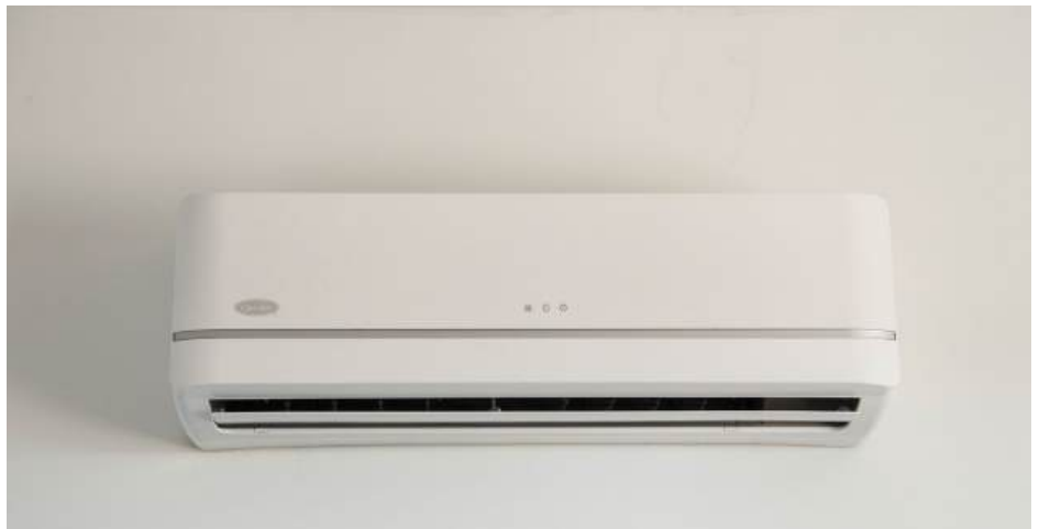
Installing a mini-split system can provide several benefits, but the capability to regulate temperatures in specific rooms or areas of the home is the most attractive feature. Photo Source: Dennis Schroeder, NREL.
