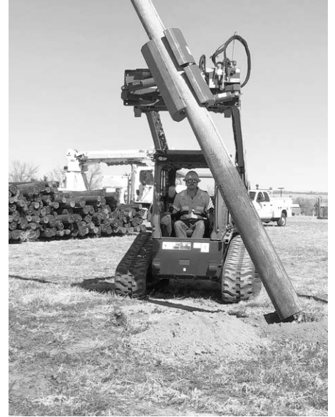
Lineman Bryson Fogg sets a pole for MCREA’s new training yard.
