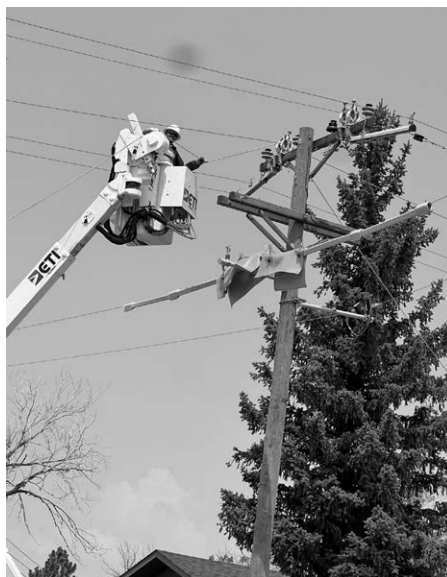
▲ A K.C. Electric lineman works on replacing power line in Hugo.
