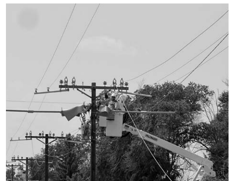
▲ Linecrews in Hugo install aluminum conductor.
